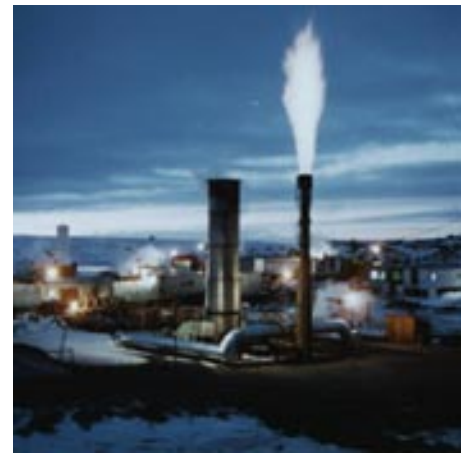
( E&TR July–August 1989) The Rocky Mountain underground-coal-gasification test facility near Hanna, Wyoming. There we investigated ways to extract energy otherwise not exploitable. Coal was partially burned underground, and the gas produced could be upgraded to pipeline quality or used as a synthesis gas for liquid fuels.
