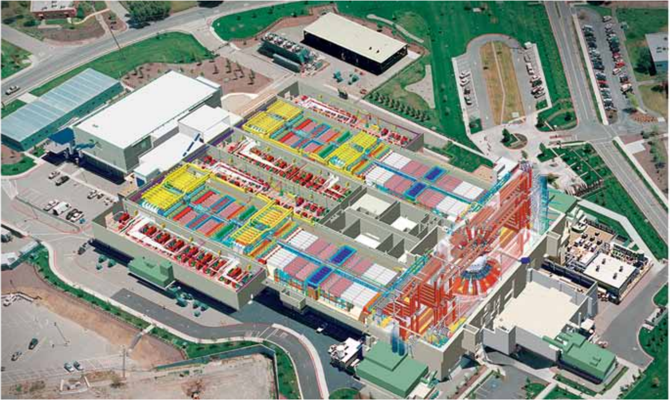
(above) The building housing the 192-beam laser and its target chamber is the size of three football fields. (below) Each of NIF's two identical laser bays has two clusters of 48 beamlines, one on either side of the utility spine running down the middle of the bay.
