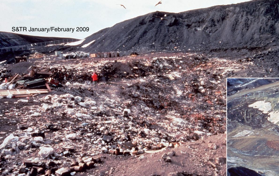
During his time in Antarctica, Allen Macenski managed the cleanup of a 5-acre legacy waste dump at McMurdo Research Station. (Inset) The waste was excavated, segregated, containerized, and shipped off the continent, revealing a more pristine landscape.
