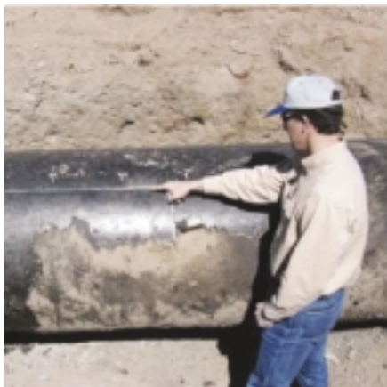
A Pacific Gas & Electric worker points to one of the discovered leaks in the exposed pipe.
