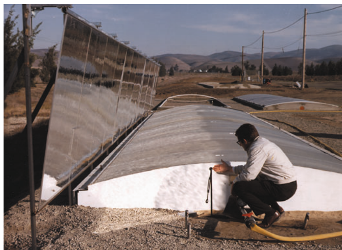
In the 1970s, the Laboratory explored the feasibility of using shallow ponds to store solar energy to produce domestic heat and run chemical processes.
