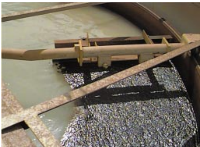
Figure 3. Contaminant floating on water in the dissolved-air-flotation tank (at lower right). Dissolved air forms bubbles that capture and lift free-product contaminant to the surface of the separator.
