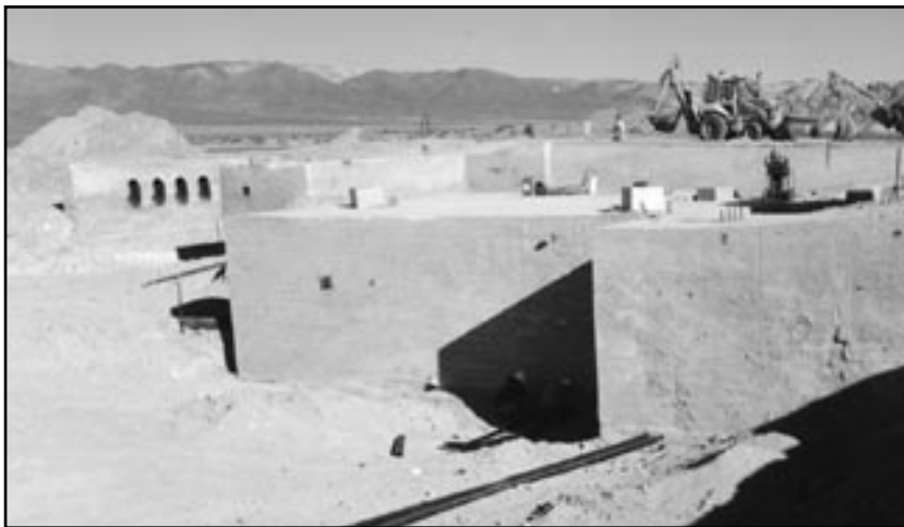
A major construction project at the Nevada Test Site, BEEF (Big Explosives Experiment Facility) is using underground bunkers from atmospheric tests (seen unearthed here) as a base facility for large-mass hydrodynamic diagnostics experiments.
