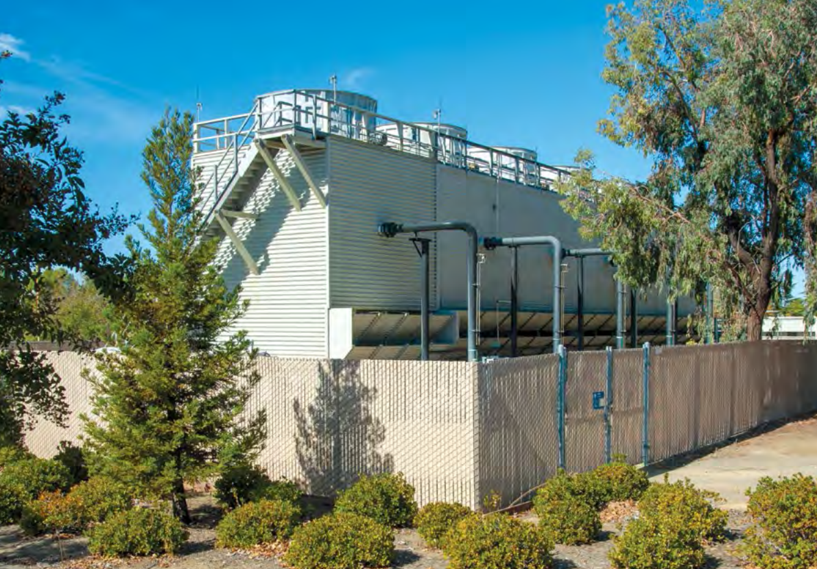
Cooling towers, which feed water to the air-conditioning systems for the Laboratory's high-performance computing facilities, account for about 45 percent of the total water consumption at Livermore's main site. (Photograph by Lee Baker.)
