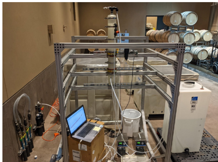
CO 2 off-gas from tanks of fermenting wine at Continuum, a Napa Valley winery, travels through plastic tubing and into the bottom of Livermore's absorber tower (center). Liquid solvent from the square container (right foreground) flows through the absorber packing.
