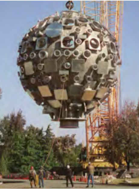
In June 1999, after careful preparation, a rotating crane hoisted NIF’s target chamber and gently moved it to the facility’s target bay, a breathtaking event that took only about 30 minutes to complete.
