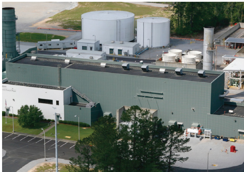
The compressed-air energy storage (CAES) facility at Alabama's McIntosh Power Plant is already using CAES in generating renewable energy. The Earth Battery would use some of the features of CAES. (Photo courtesy of PowerSouth Energy Cooperative.)
